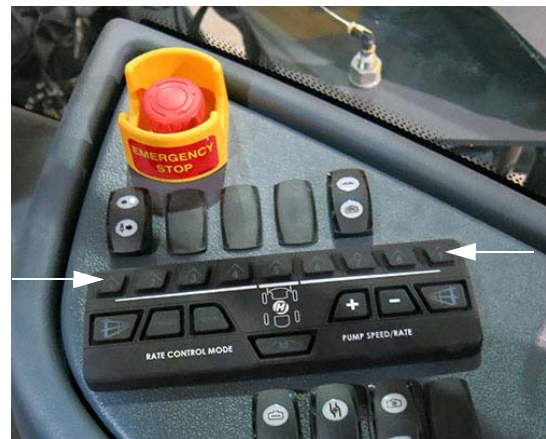
Boom Solution Valve Switches - Sections 1 and 9 (Located on the side console) -Typical View
