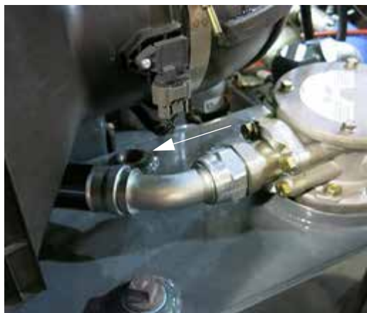
Breather Cap Removed -Typical View
