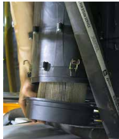
Filter Removal -Typical View
