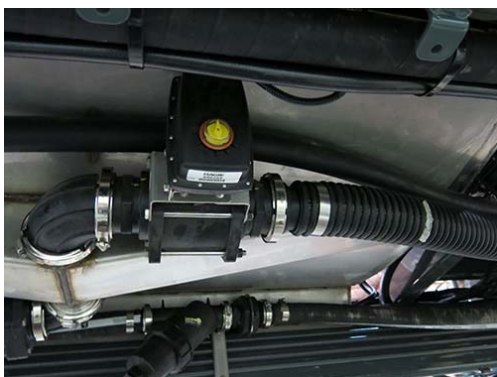
Solution Tank Valve -Typical View
