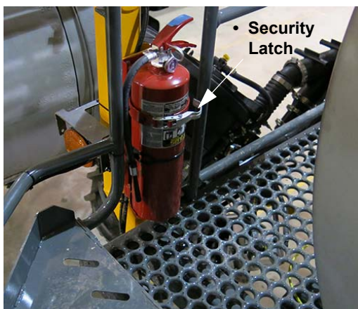
Fire Extinguisher (Located along the catwalk on left-hand side of machine) -Typical View
