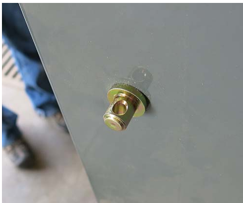
Hanger Pin Installation -Typical View
