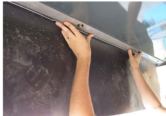
Brush Curtain Installation -Typical View
