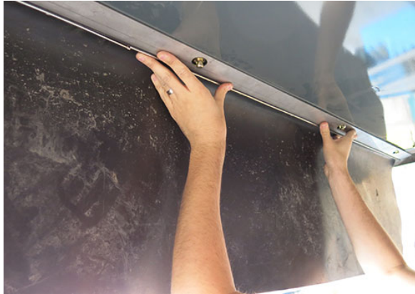
Brush Curtain Installation -Typical View
