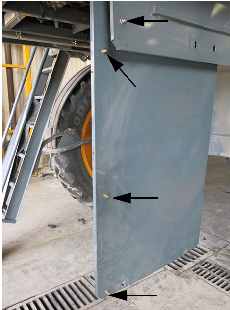
Hanger Pins (Install pins onto Panels 4, 5, and 6) -Typical View
