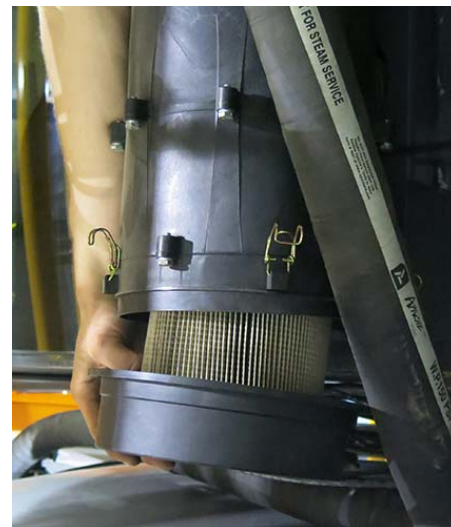
Filter Removal -Typical View
