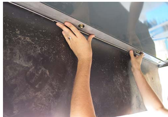
Brush Curtain Installation -Typical View
