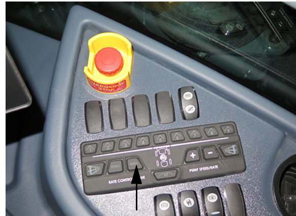
Manual "MAN" Rate Control Switch (Located on the side console) -Typical View
