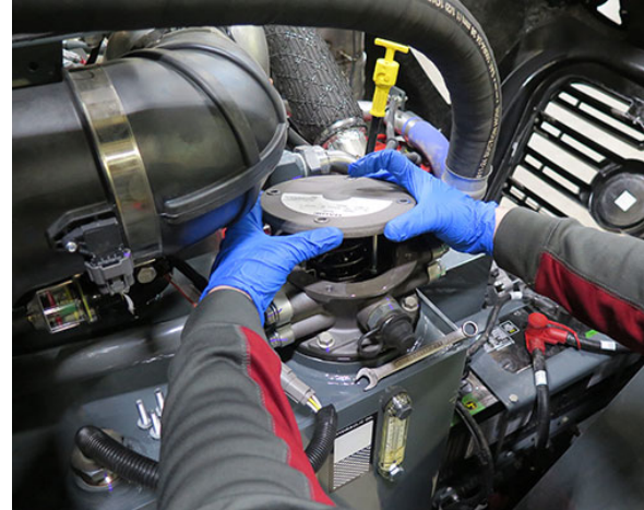
Filling Tank Through Hydraulic Return Filter Housing -Typical View
