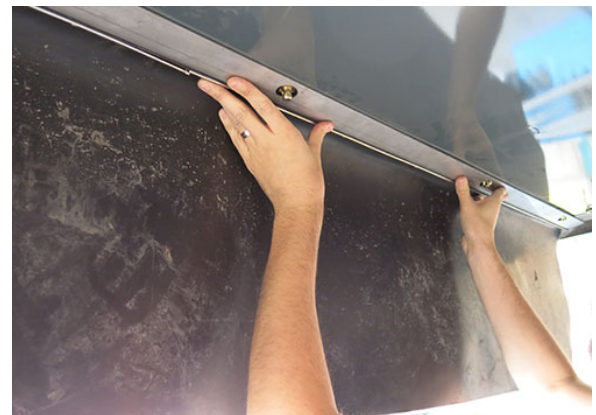
Brush Curtain Installation -Typical View
