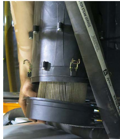
Filter Removal -Typical View
