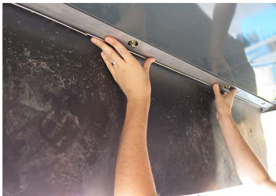
Brush Curtain Installation -Typical View
