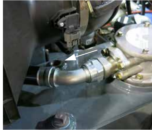
Breather Cap Removed -Typical View
