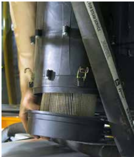
Filter Removal -Typical View
