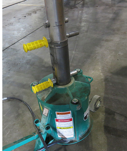
Lock Pin Installation -Typical View
