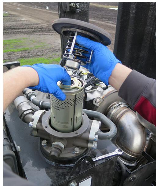
Return Filter (Located inside filter housing) -Typical View
