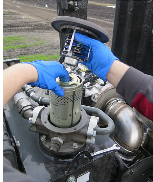
Return Filter (Located inside filter housing on top of hydraulic oil reservoir - open hood to access) -Typical View
