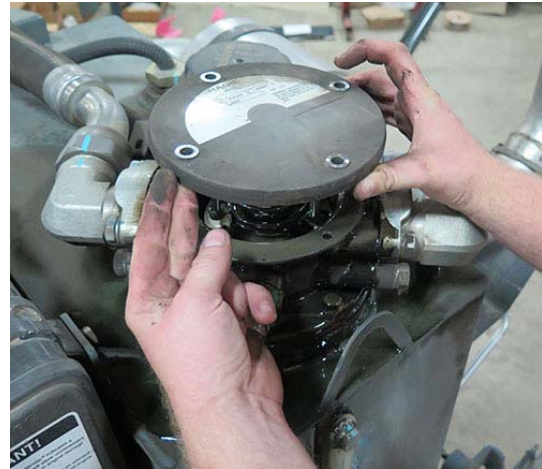
Filling Tank Through Hydraulic Return Filter Housing -Typical View
