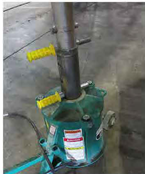
Lock Pin Installation -Typical View
