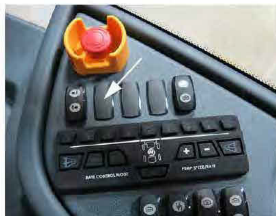
Night Spray Switch (Located on the side console) -Typical View
