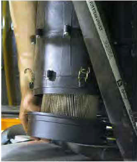
Filter Removal -Typical View
