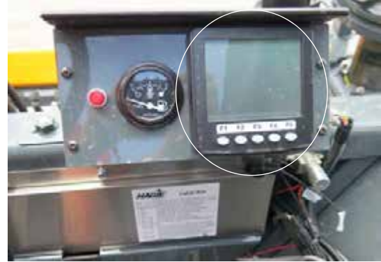
CANtrak Engine Monitor (Located near the front of operator's station) -Typical View
