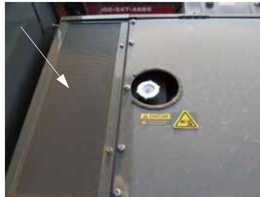
Top Grille Screen (Remove two radiator panel bolts and panel to access) -Typical View
